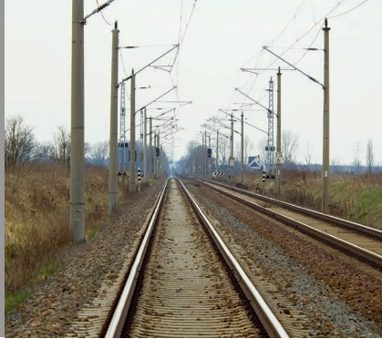
Concrete poles with railway overhead lines; © Uwe Bumann - Fotolia
